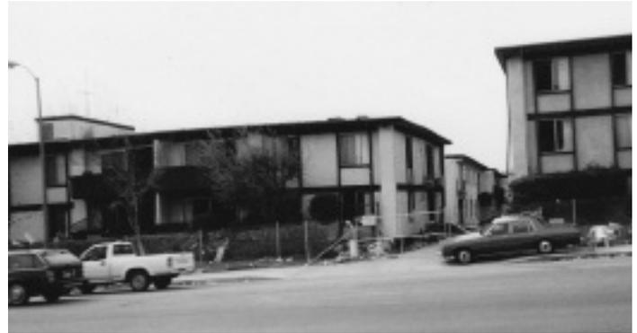
*The apartment building on the left, severely damaged in the 1994 Northridge Earthquake, looks almost normal, until you look closer and realize that the entire first (soft) floor collapsed, reducing it to a two-story building.*
